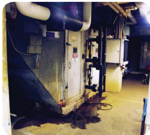
Aluminum units (left) provide a long life and high return on investment; steel units (right) are prone to degradation, creating environments that lead to infectious control issues.
