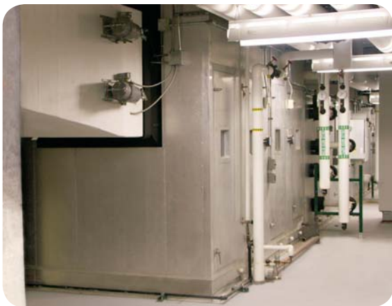
Aluminum units (left) provide a long life and high return on investment; steel units (right) are prone to degradation, creating environments that lead to infectious control issues.
