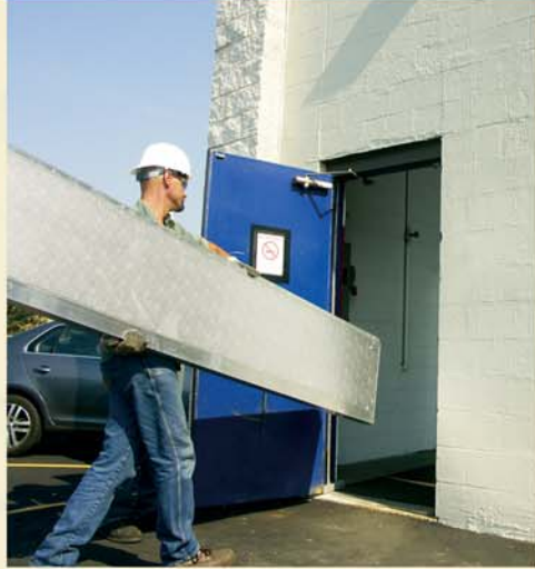
Lightweight, aluminum components are easily transported on site through any building access and are staged for rapid assembly.
