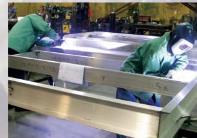
SiteBilt components are precision fabricated with the same care as factory units.
