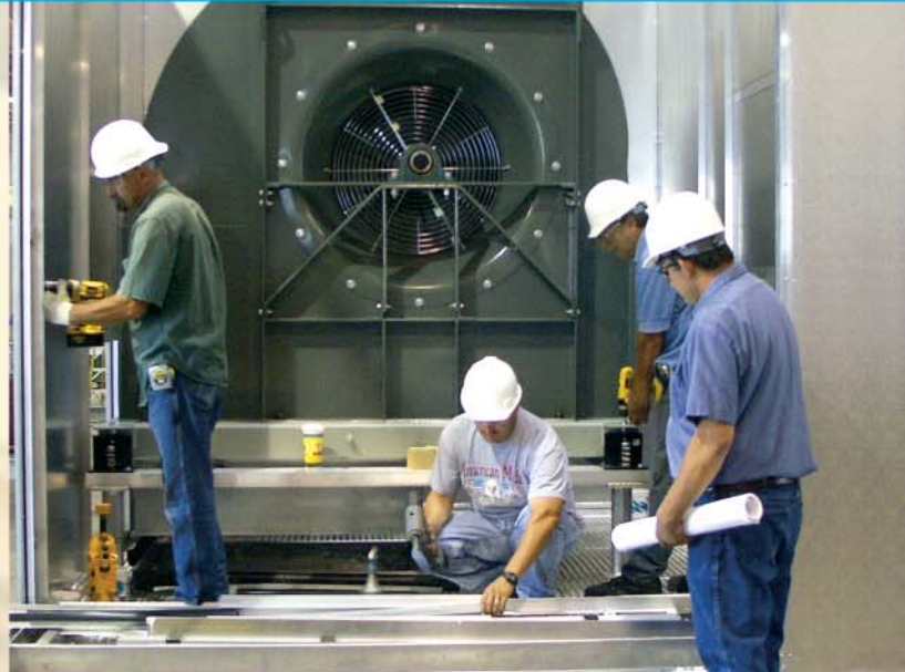
Work goes fast with local contractors, directed by Air Enterprises project supervisors.
